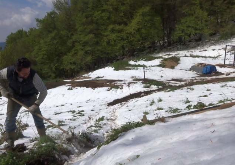
Fig.065 Screenshot showing me attempting to clear a path to reach the building site of my ark in the alps. The physical work is made most strenuous by the actual remoteness of the site. There are barely any roads to reach it and it is completely disconnected from the grid. All the heavy steal and equipment had to be carried individually.
